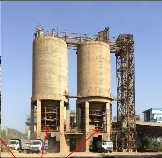
Closed body truck with modified opening for Ash filling through Telescopic spout arrangement
